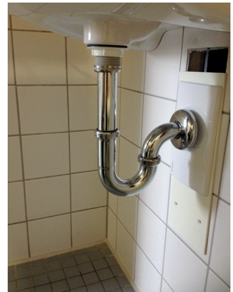
Figure 2: S-shaped siphon trap.
